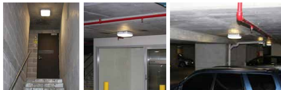
From left: Chamaeleon installations in fire stair, car park lift lobby and car park parking bays
